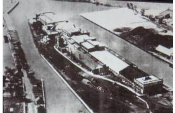
Manufacturing on the Port Hope Pier in 1951.
